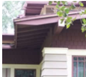
Exposed Rafter Tail
