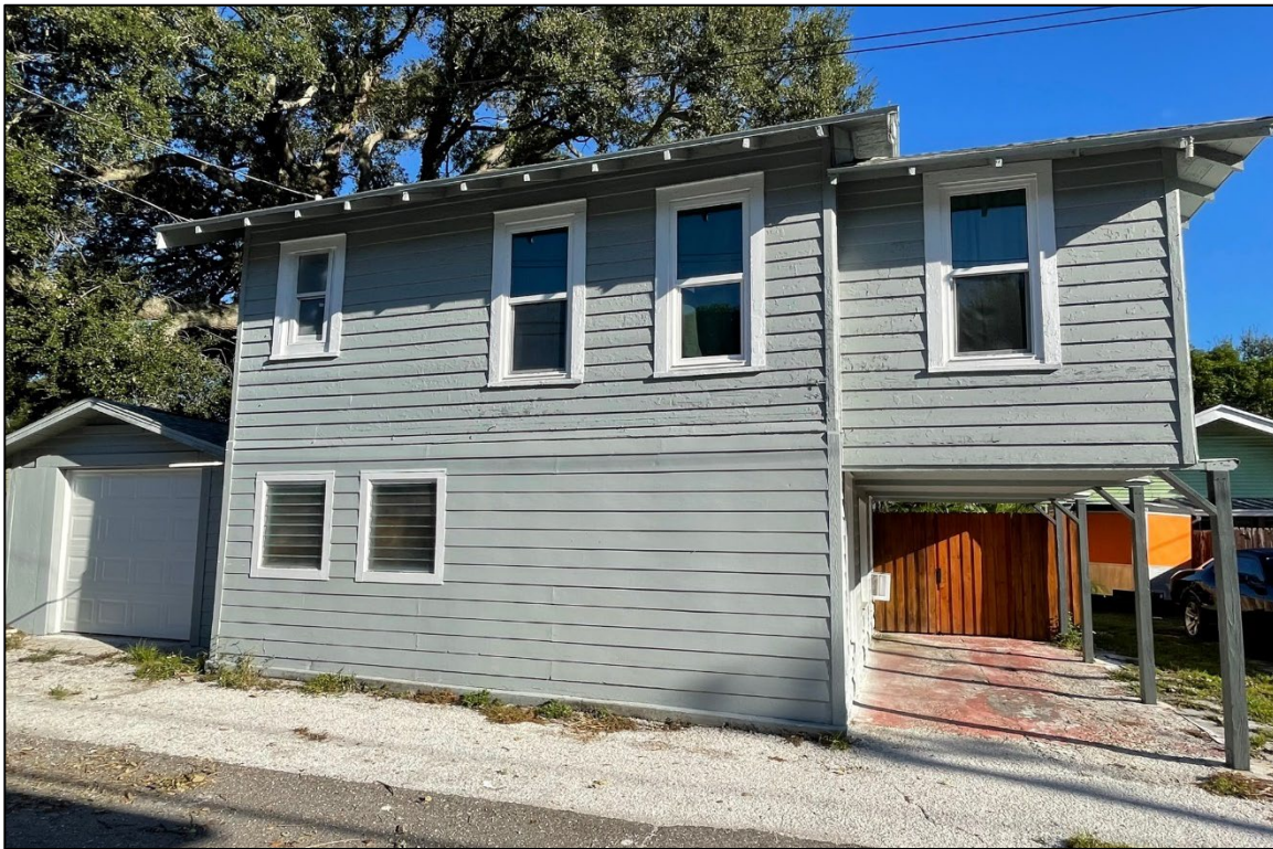
Figure 5: Photograph of rear accessory building, taken from alleyway.
