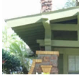
Exposed Rafter Tail
