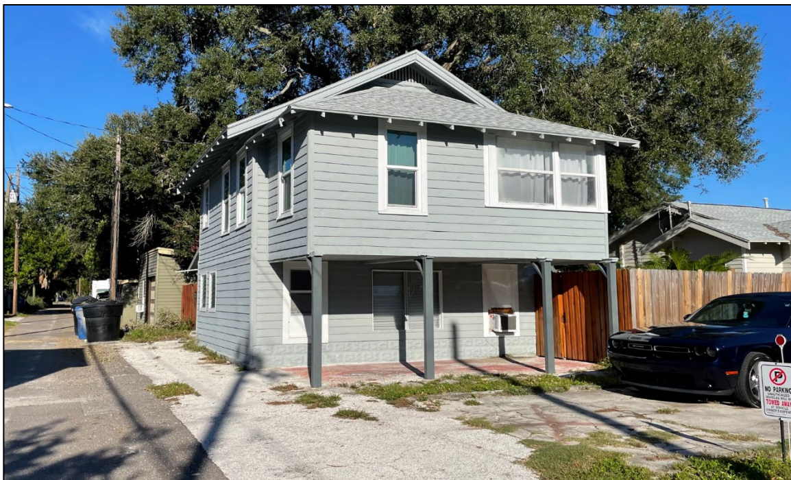
Figure 5: Photograph of rear accessory apartment building with newly installed sash windows.
