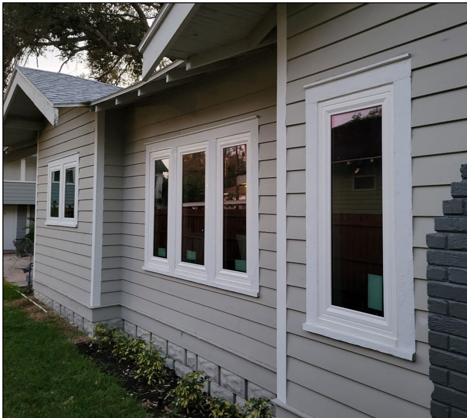
Figure 3: Close-up photograph of east elevation of installed picture windows.
