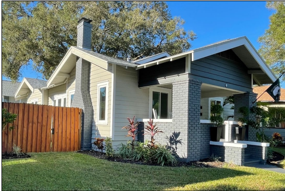
Figure 2: Photograph showing the installation of the unapproved picture and horizontal slider windows and the newly installed wood siding.
